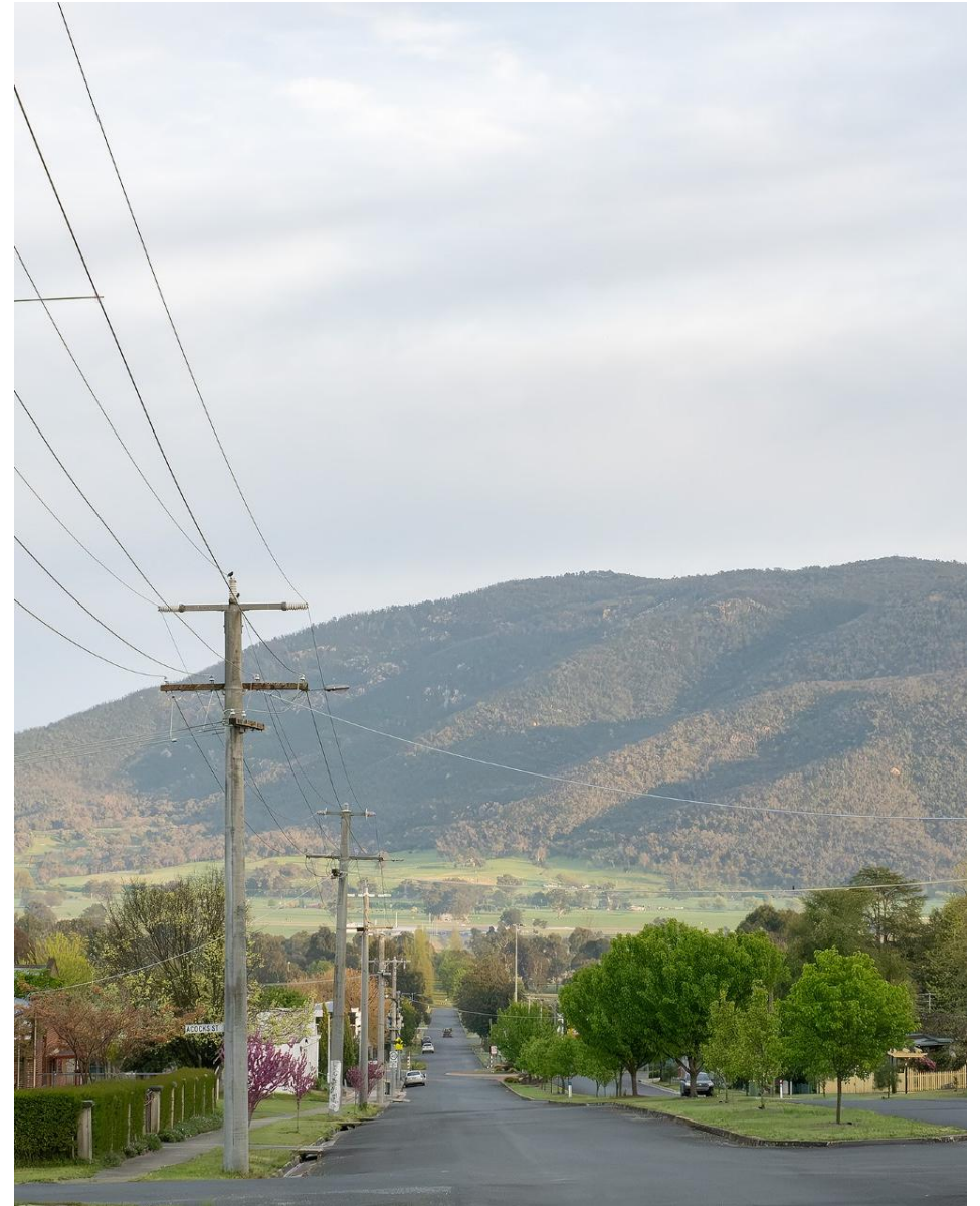
Corryong (VIC), location of an AusNet Services owned Microgrid
